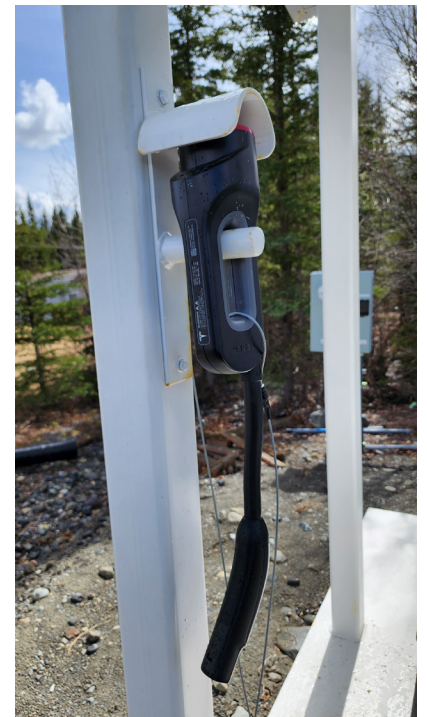
A NACS adapter installed at a charging station in Glennallen is attached by a metal cable. Photo courtesy AEA.
